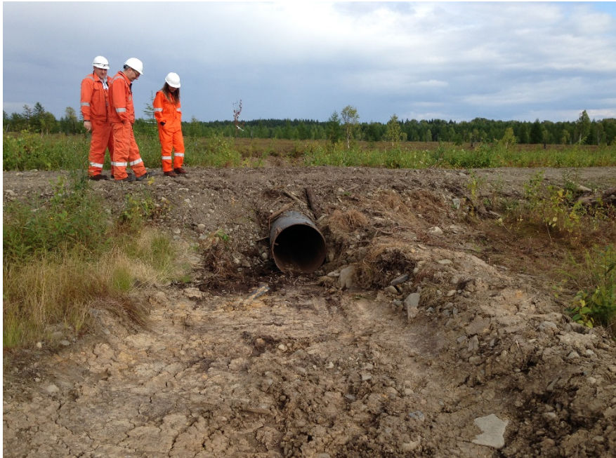
Photo 1. Newly installed culvert
