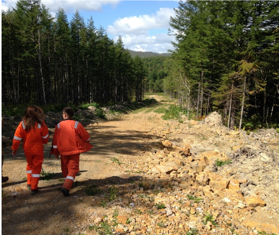
Photo 2. Recently cleared access track to BS4
