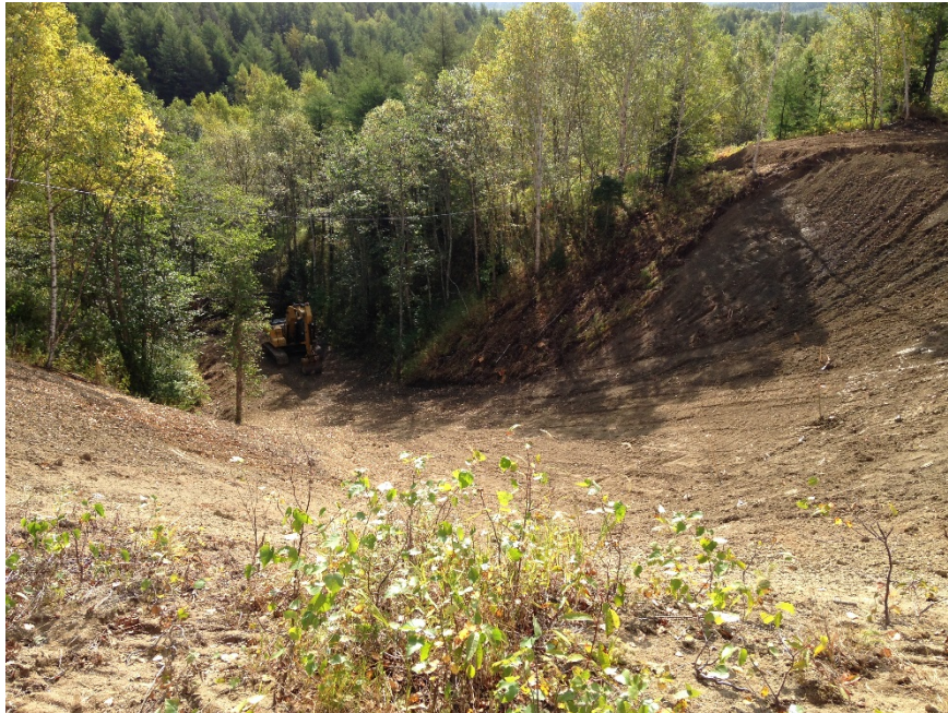
Photo 1. Re-profiled slope – ready for installation of netting
