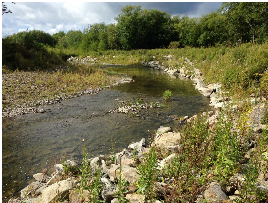
Photo 1. Rock armour placed 4 years ago, showing good vegetation regrowth in cracks
