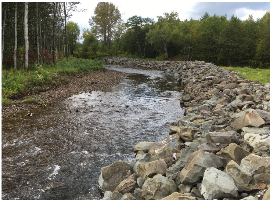
Photo 1. Stone rip-rap erosion protection
