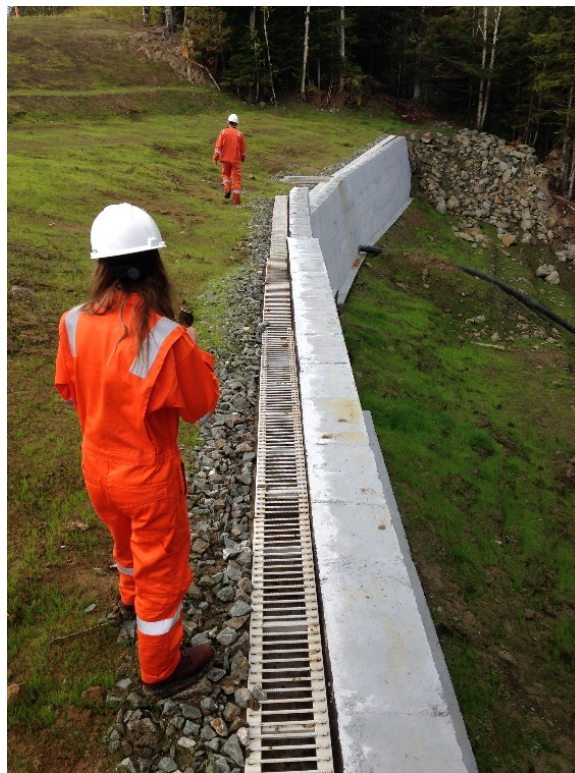
Photo 1. View of reinforced concrete retaining wall, outflow drainage pipe and recently reseeded soil surface.
