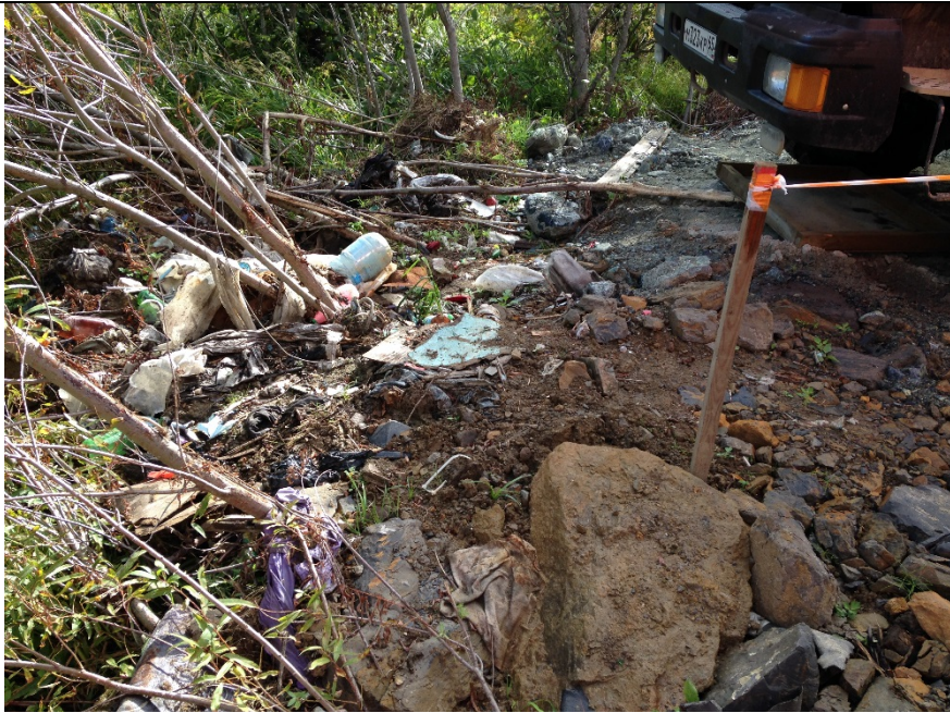
Photo 3. Fly-tipped rubbish that has been incorporated within the filled base of the temporary work camp.
