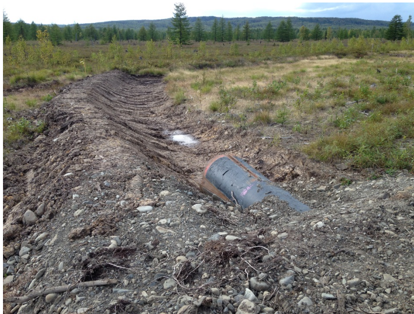
Photo 2. New culvert, low bund and shallow ditch
